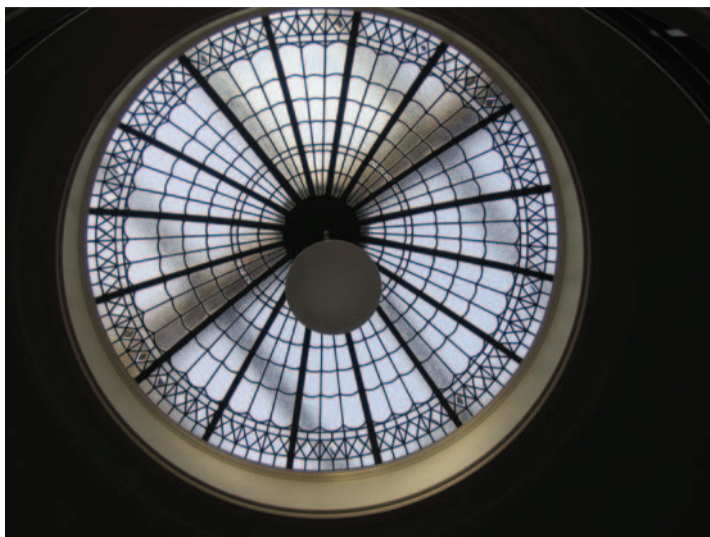
View of the cupola from the reception area, Sainsbury Logan & Williams building. Image source: Sainsbury Logan & Williams Archive.
