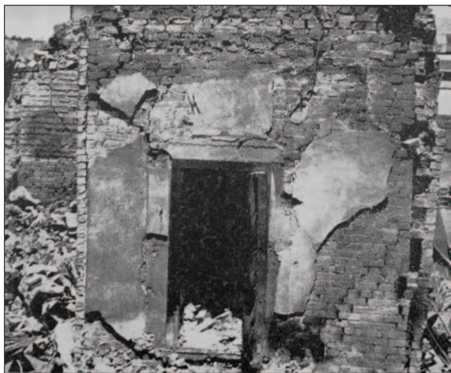
Bank of New Zealand strong room that was no so fortunate. Image source: Geoff Conly, Hawke's Bay Before and After: The Great Earthquake of 1931: An Historical Record , Daily Telegraph , Napier, 1981, at page 124.
